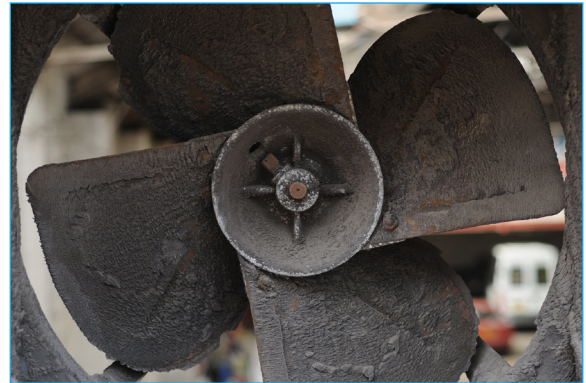
Figure 9: A dirty ventilation fan.
