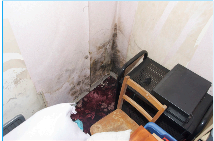
Figure 12: Mould growth and dampness.
