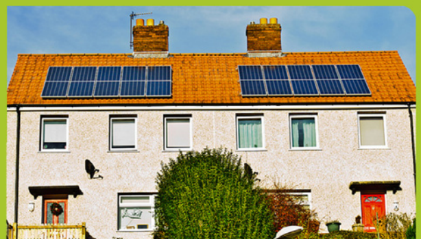
Bron Afon has fitted solar PV panels to 771 homes and 5 retirement homes in Torfaen, helping tenants to stay warm
