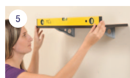
Finally, install and level the shelf
