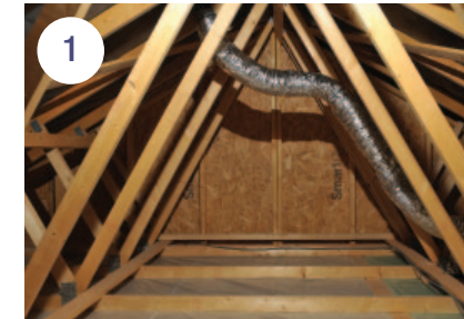
OSB sheathing on the gable wall
