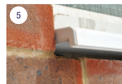
Movement gap under window
