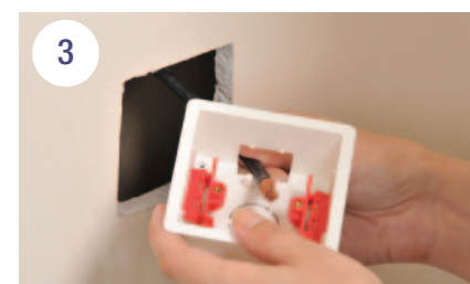
Pull the cable through the back of the box
