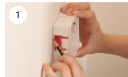
Mark the outside of the box on the wall
